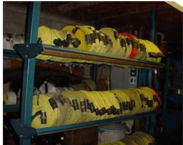
**Indoor hose storage**—Fire hose life can be extended when properly maintained and stored, and will provide dependable service on the fireline. Storage racks can be constructed to provide a neat, well-ventilated hose storage area. There are other methods that can be “homemade” and just as practical.
