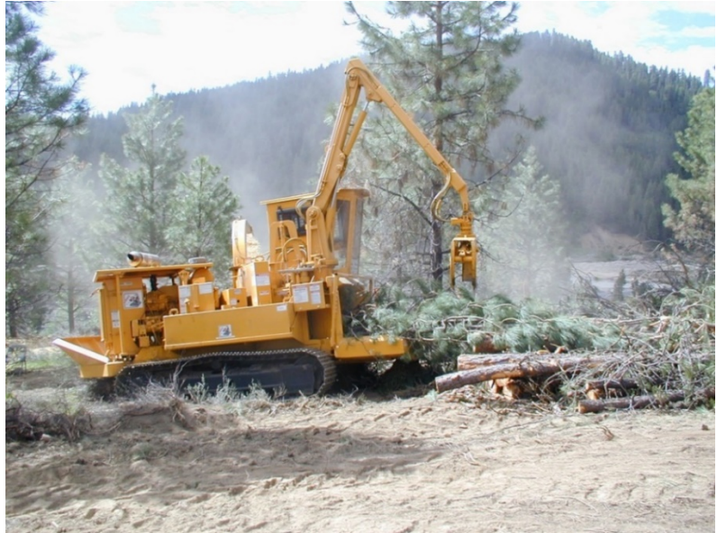
Figure 4.2.2. Mechanical processing of biomass.
